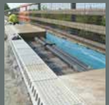
Combined Kerb, Bridge & Sub-Surface Drainage
