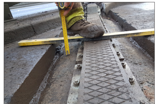
Checking level after joint is installed against adjacent road surface
