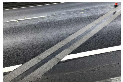
North bound, Auchinlay Rail Bridge - Completed installation of T-Mat 30 expansion joint
