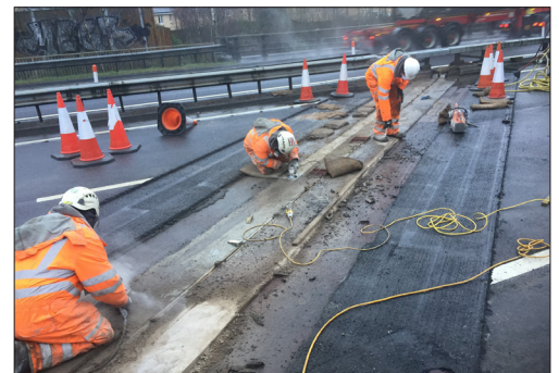
Installation of expansion joint sub-structure
